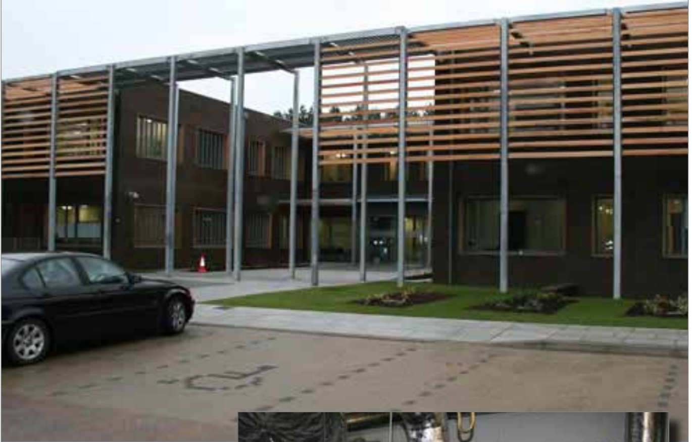
Corporate Headquarters for client VolkerFitzpatrick in Hoddesdon. Below: circulating pumps for GSHP system and incoming flow and return pipework form the closed loop ground array.
