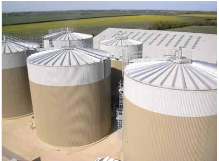
The integrated Anaerobic Digestion process uses food waste and pig slurry to create clean energy and bio-fertiliser.
