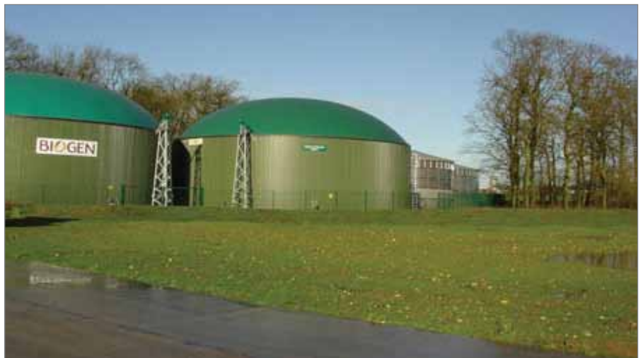
The integrated Anaerobic Digestion process uses food waste and pig slurry to create clean energy and bio-fertiliser.
